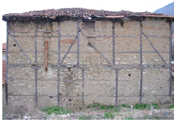
Fig. 8 - Rear façade of a 19th c. traditional house in Florina.
