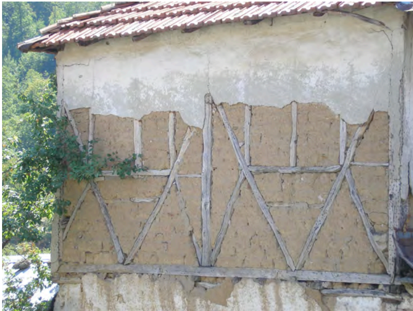
Fig. 10 - Timber frame construction of a house in Alona, Florina area.
